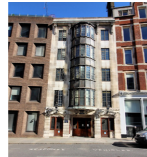
Fig. 34 Snowhill Police Station Grade II | Early C20
