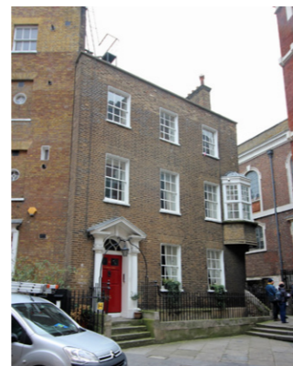
Fig. 45 The Rectory Grade II | Late C18
