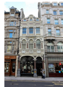
Fig. 49 29 Fleet Street Grade II | Late C19
