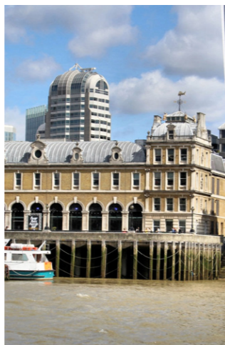
Fig. 40 Billingsgate Market Grade II | Late C19
