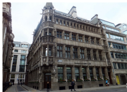
Fig. 50 13 & 15 Moorgate Grade II* | Late C19
